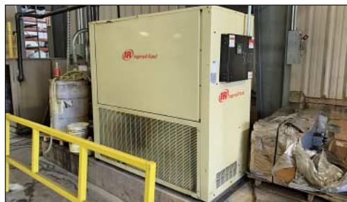
Ingersoll Rand Refrigerated Air Dryer
